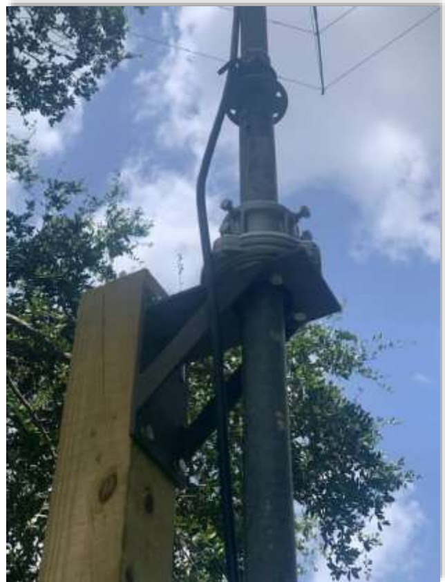
Thrust bearing and mounting bracket as installed at previous QTH.
