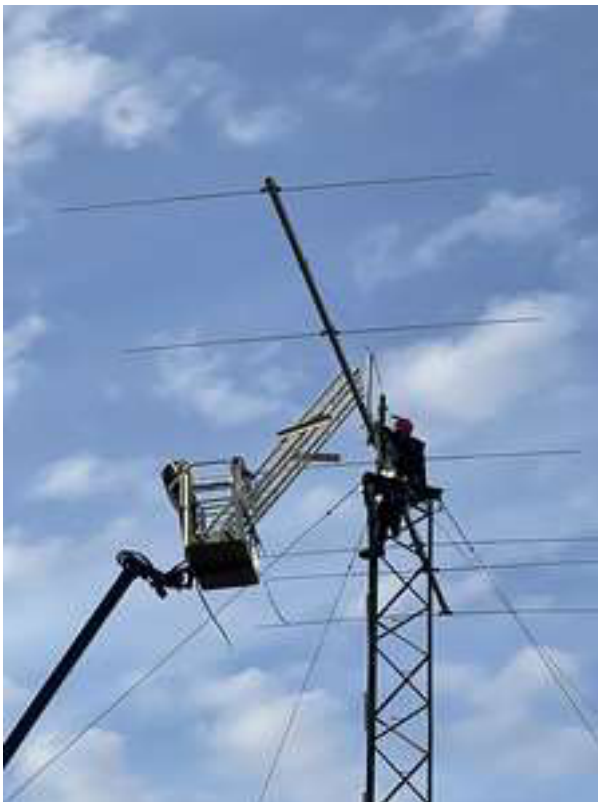
Benni atop the tower with the new 2el West-facing 40m Yagi.
