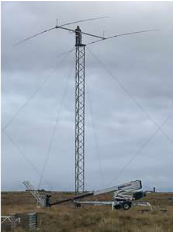
Benni atop the tower with the new 2el West-facing 40m Yagi.
