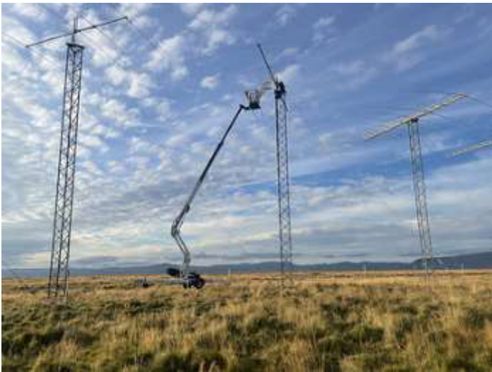
West-facing 10m Yagi going up with help of a man-lift.
