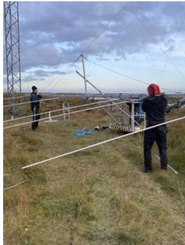
Benni and Gudmi preparing the East-facing 15m Yagi for installation.
