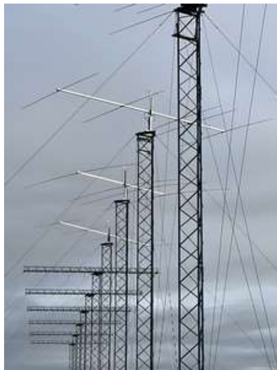
West-facing 10, 15, 20m Yagis and SuperDARN Log Periodic antennas, all on 50 ft towers.
