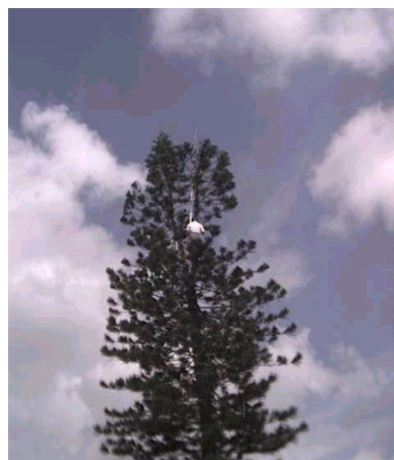
FCGer Bob N4BP installing a mast at the top of an 80 ft. pine tree in Bruce W4OV's front yard. A pulley has been installed at the top to hoist various loop antennas up and down. Watch out for Bruce in next season's 160 meter contests, where he's hoping that a loop antenna with this kind of apex elevation will be very effective.
