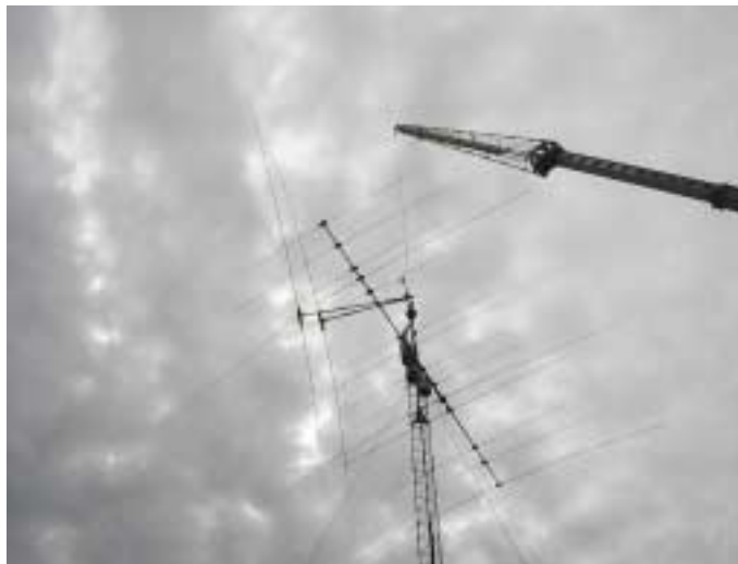
Removing bent mast and folded up XM-240
