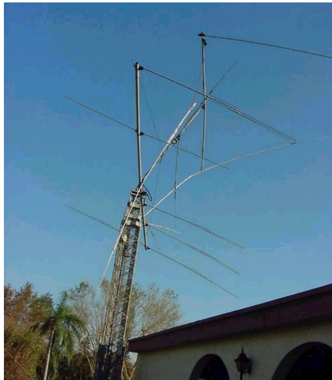
N8PR - Hollywood One Tower and Antennas
