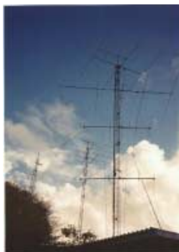
USA Tower - Rotatable CL-33 at top, 5 el 20 , 2 3el 10's, and a 6 meter beam at top.
