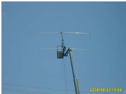
Beams on 20 and 6 on hydraulic lift at K4F
