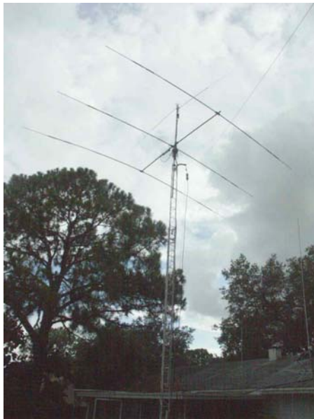
W4LT Antenna and Tower: EZ-Way HDX-40 tilt over telescoping tower, Alliance HD73 rotor, HyGain Thun- derbird 3 Junior, Dual band 40/80 dipole with Reyco Traps. W2DU Current Baluns, 30 meter mobile whip dipole mounted above
