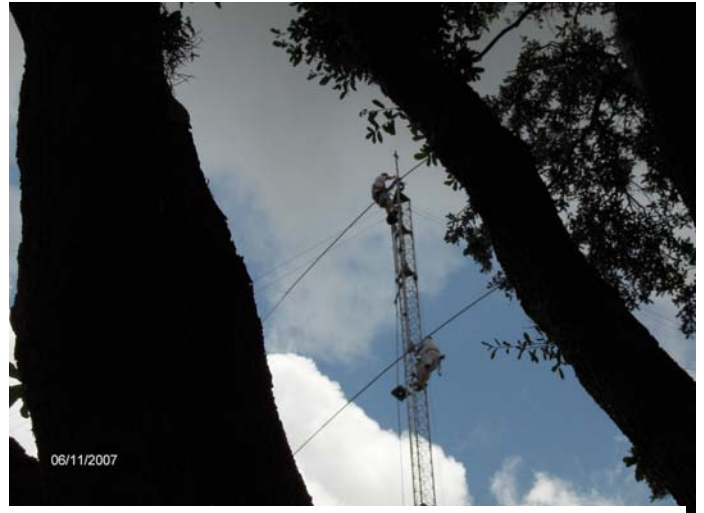
The first 40 meter element disconnected and getting ready to go down the tower
