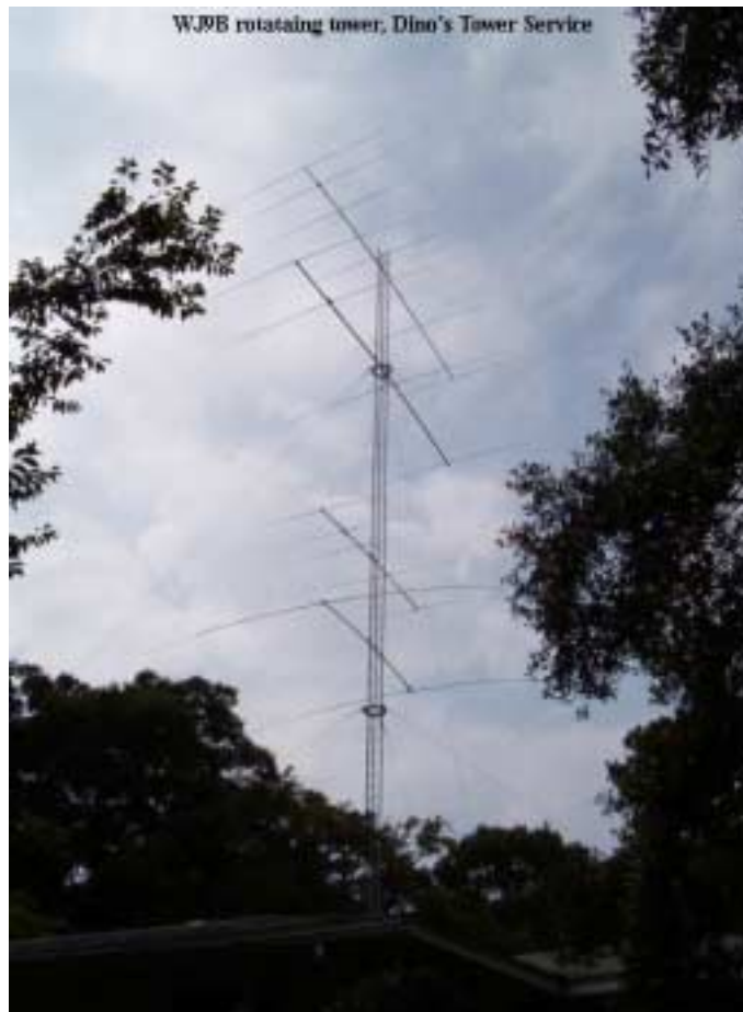
WJ9B has moved in! Will just got his new tower installed in Gainesville. Antennas, top to bottom include M2 15M6, M2 20M4, Hygain 105CA, Cushcraft 40-2CD, all on a K0XG Rohn 55 rotating base.
