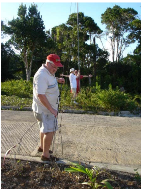
K1XX building 2 element 40 meter loops on 50 ft fiberglass masts.
