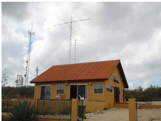
Radio Huis in Rincon, Bonaire. C31 on the front tower, and 2el 40 and C3 on the back 90' tower. Commercial radio service on the hilltop in the background.
